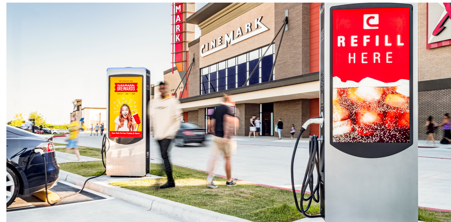
Volta charging station at Cinemark Theatres in McKinney, Texas, a STORE-owned property.
